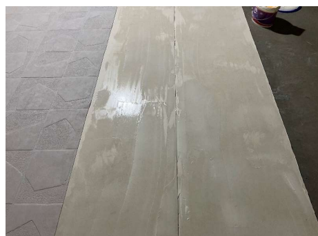
photo: during bonding the wall covering on the plasterboard
