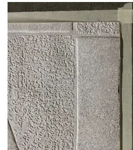
photo : detail of the joints between the multiple bands of the wall covering and the side edges, covered with a non sound absorbing tape
