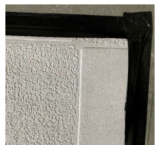
photo : detail of the joints between the multiple bands of the wall covering and the side edges, covered with a non sound absorbing tape
