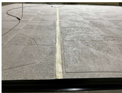
photo : detail of the joints between the multiple bands of the wall covering and the side edges, covered with a non sound absorbing tape
